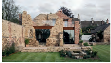
Gretton Parchment Works incorporated into new extension.
