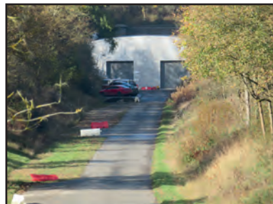
The tunnel's southern portal is obscured by the new building.
