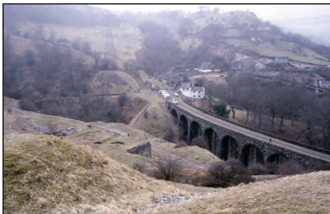
The Nantdyar viaduct © Geoff West 1986
