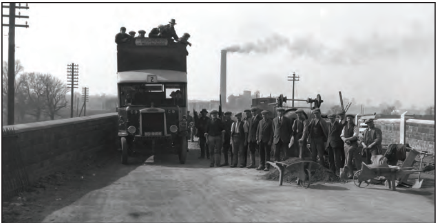
Finedon Road bridge
