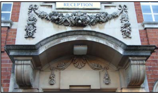
Stone detail on the former Victoria Works.
