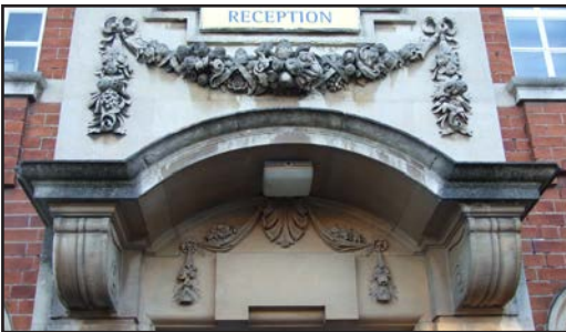
Stone detail on the former Victoria Works.
