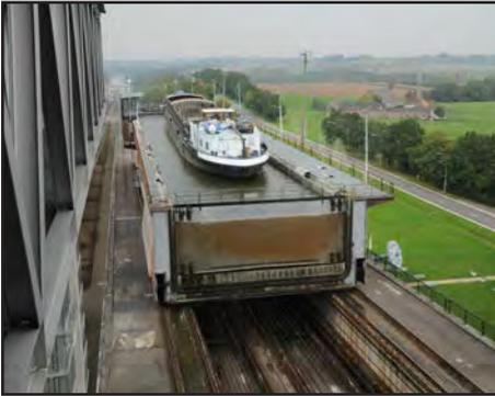
Shown on the left each caisson, 91m long and 12m wide, travels longitudinally on a pair of rails on each side of the incline supported by 236 wheels 700 mm in diameter arranged on 59 axles. Depending on water levels in the canal, the depth of water in the caisson varies between 3m and 3.7m; the total weight of the caisson varies between 5,000 tonnes and 5,700 tonnes. A counterweight of 5,200 tonnes also travels on four rails that are set between, and at a lower level than,
