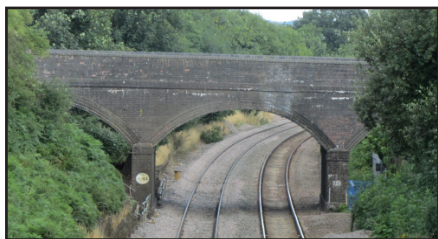
Bridleway bridge - Before and After
