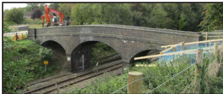
Footpath bridge - Before and After
