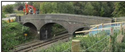
Footpath bridge - Before and After
