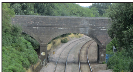
Bridleway bridge - Before and After
