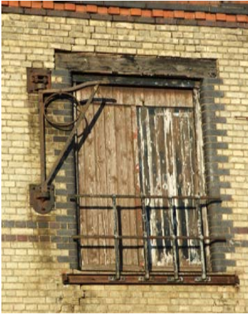
Loading door on the Ernest Chambers factory
