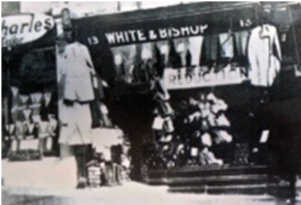
A photograph showing the original shop front as can be seen on their web-site.
