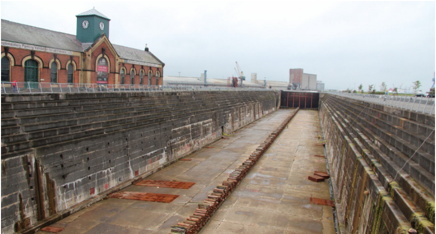
The Thompson Dry Dock and Pump-House at Belfast Shipyard which was built for the Titanic in 1911.
