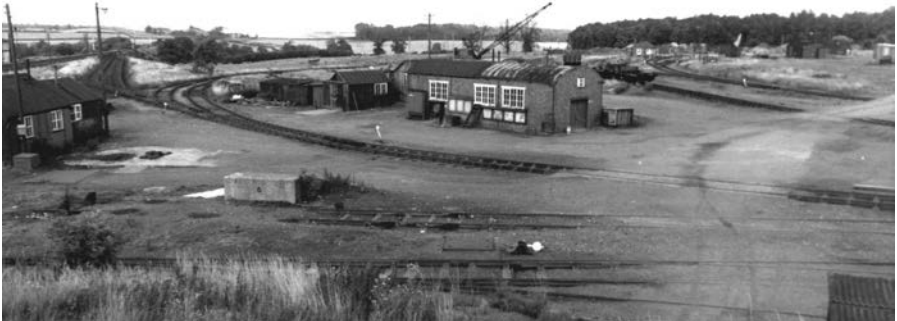
Quarry buildings and layout just after activities had ceased. Taken just east of the bridge over the BR line.
