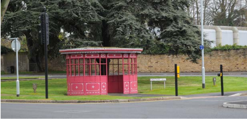
Kingsthorpe restored tram shelter
