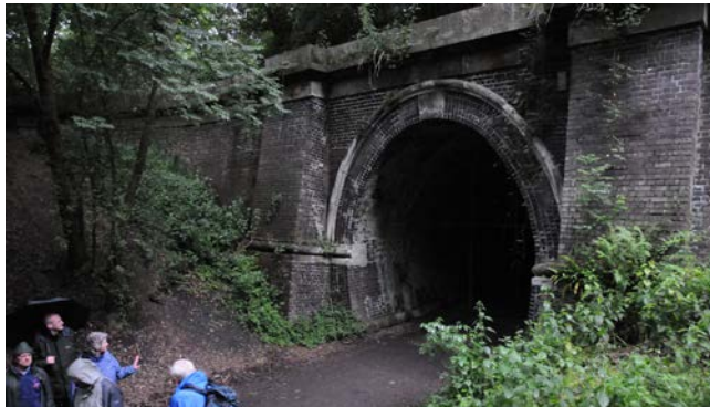
Exiting the tunnel
