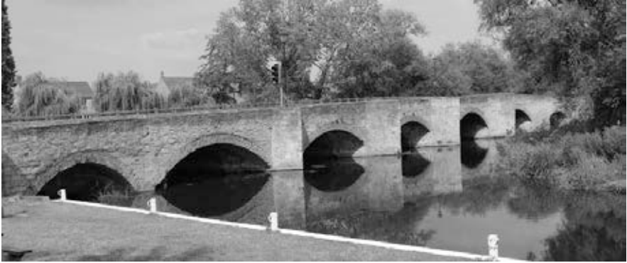
The medieval Nine Arches road bridge over the Nene
