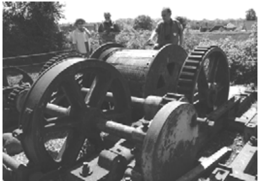
Winding gear (c) Terry Waterfield 2010
