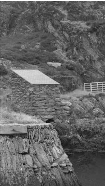
Two seater toilet
