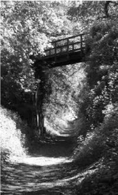
The Incline showing the Potato Lane bridge (c) Jane Waterfield 2010
