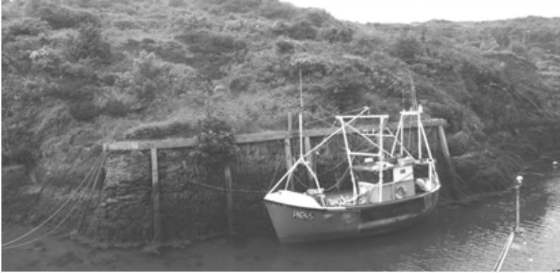
Part of the old quay
