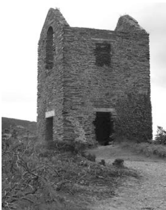
Pearl Engine House
