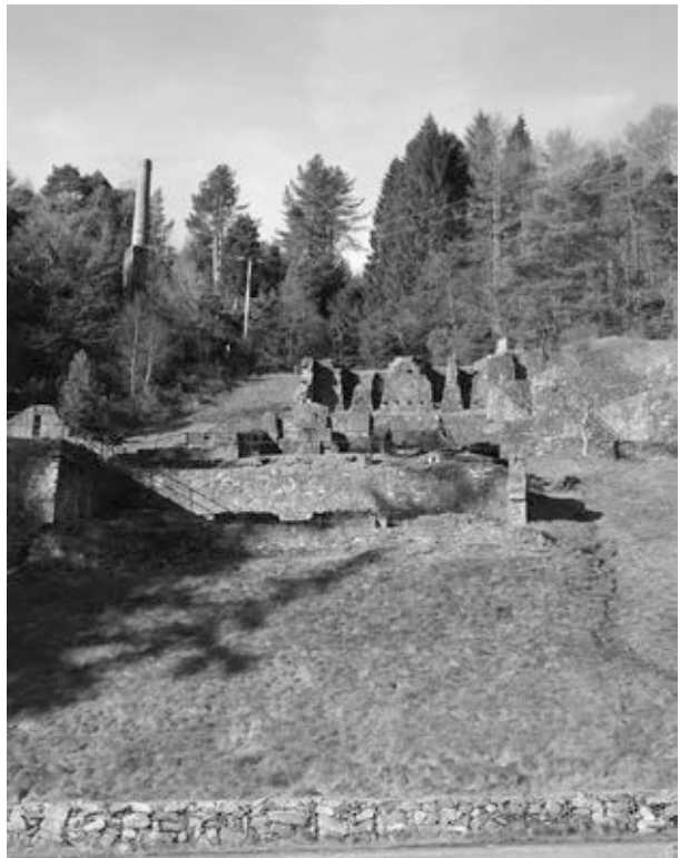
Hafna mine showing its furnace chimney
