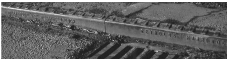
Williamson & Reynolds Iron Kerbs, Rushden – October 1977
