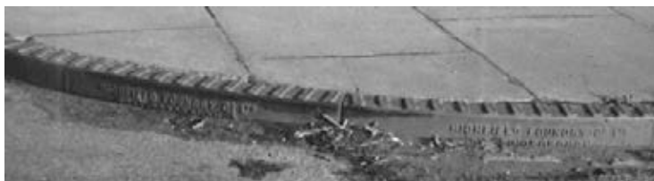
Highfield Foundry Iron Kerbs, Rushden – October 1977
