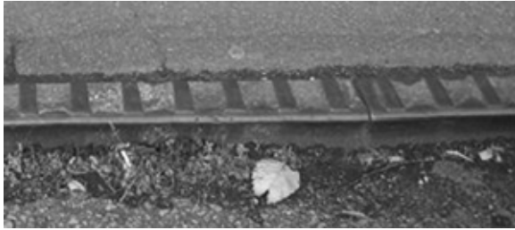
Kerbing at Wellingborough
