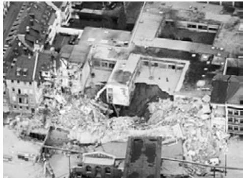
The front of the building has completely gone
