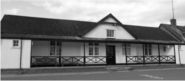
The pavilion which is built of corrugated iron.
