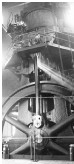
Gallows blowing engine, Kettering Furnaces.
