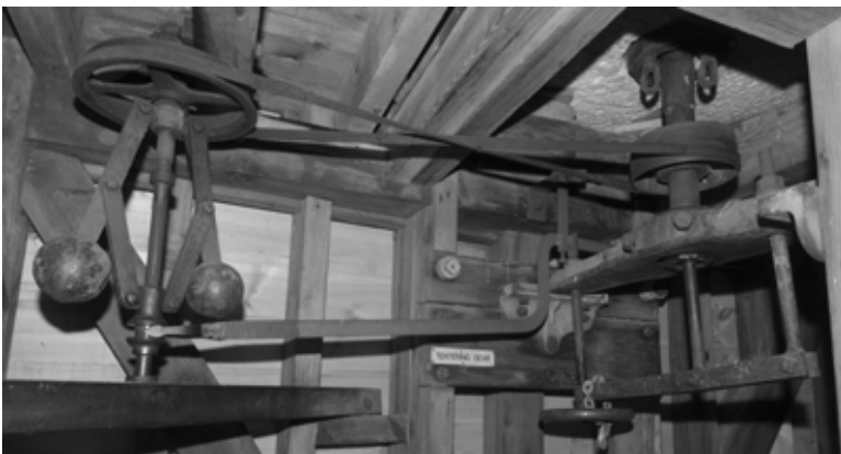
The 'tentering gear' that controls the separation of the two millstones dependent on the wind speed and hence the speed of grinding. © Tony Johns 2008
