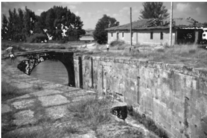
Elliptical Lock, Alar del Rey, Canal de Castella, Spain © Geoffrey Starmer collection
