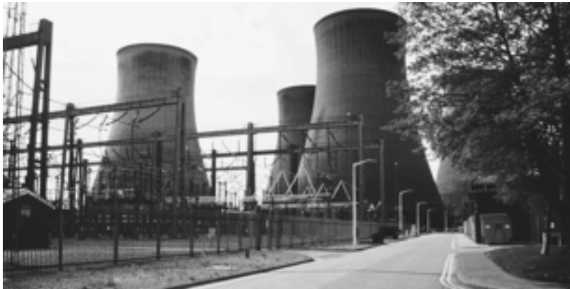
Rugeley Power Station - The chimneys and transformers.
