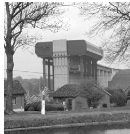
Strépy-Thieu Boat Lift. View from SW.
