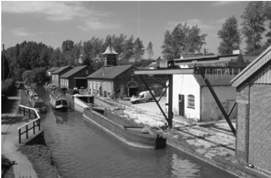
Former BWB workshops, Bulbourne. View from the SE.
