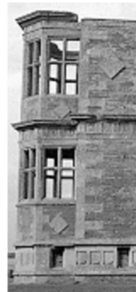
Lyveden's famous outline A combination of Weldon stone dressings and local Blisworth Limestone
